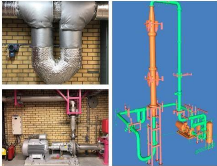
Figure 5. The EMBLA loop layout. Top left: Coriolis flow meter. Bottom left: Pump. Right: Overview.
